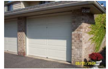
New, steel garage doors
